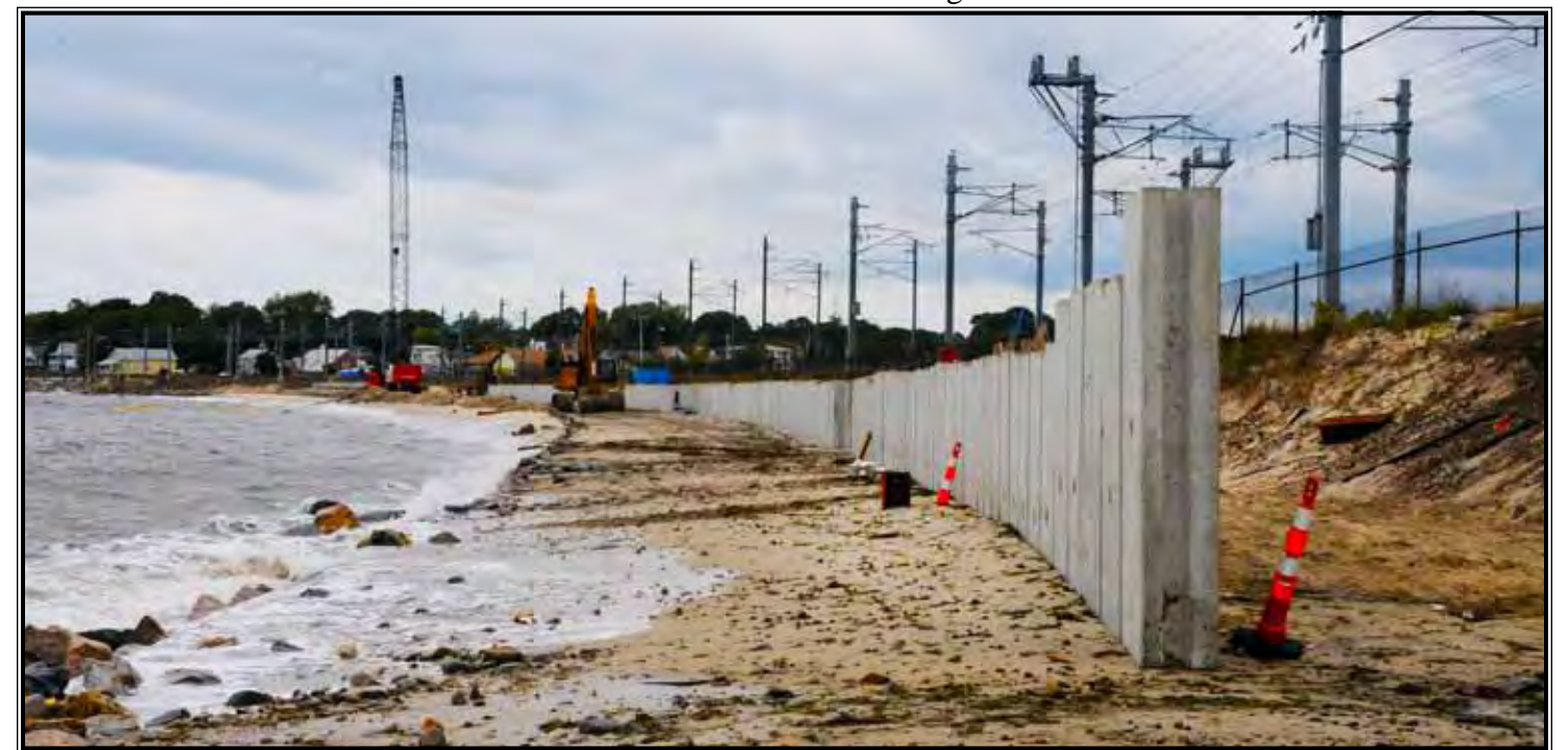
Seawall Construction Progress
