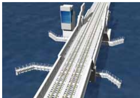
This artist's rendering of the new Niantic River Rail Road Bridge is based on the actual engineered drawings from which the bridge is being constructed. Absent from the rendering are the catenary transmission wires, poles, and their supports used to transmit electricity to the trains. Also not shown is the shoreline and new pedestrian underpass that will provide access under the western most trestle to the new Niantic Bay Overlook.
