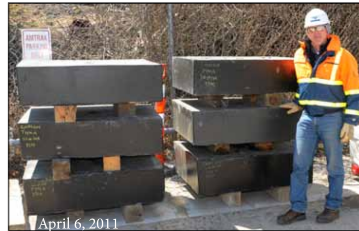
the photograph above taken April 6, 2011. These six lead ingots each weighs approximately 8,500 pounds and represent a small fraction of the Balance Plates needed for the project.
